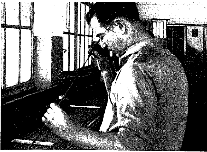
Inspecting pinion rod prior to shipment.
